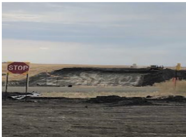
Dozer stripping (S.E) – Sf 151 – Sept 10, 2018
