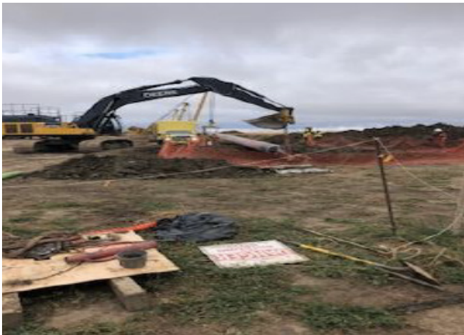
Bore being pulled – km 178+000 - Sept 14, 2018
