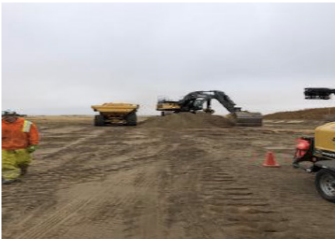
Stripping on ROW – km 164+800 – Sept 13, 2018
