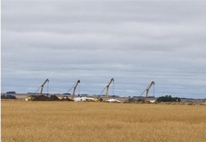
Mainline welding – km 146+076 - Sept 14, 2018
