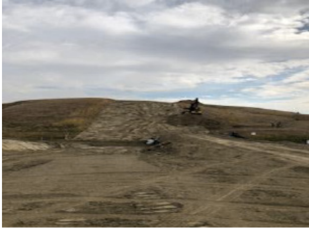
Excavator stripping topsoil – km 222+781 – Sept 10, 2018
