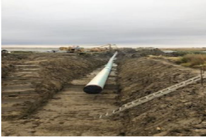
Mainline section lowered into ditch - km 165+200 – Sept 15, 2018
