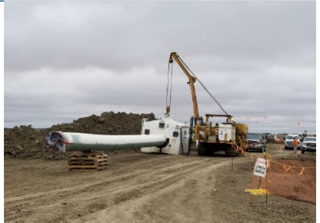
Welding Shack - km 146+076 – Sept 13, 2018
