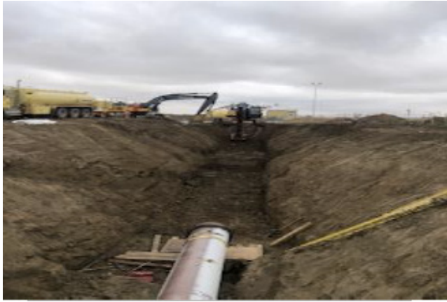
Tie in crew digging - Km 147+970- Sept 11, 2018
