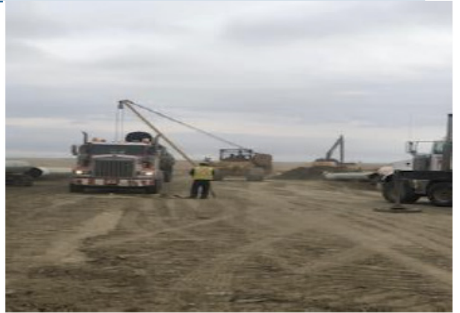
Unloading of bore casing and auger – km 222+300 Sept 15, 2018
