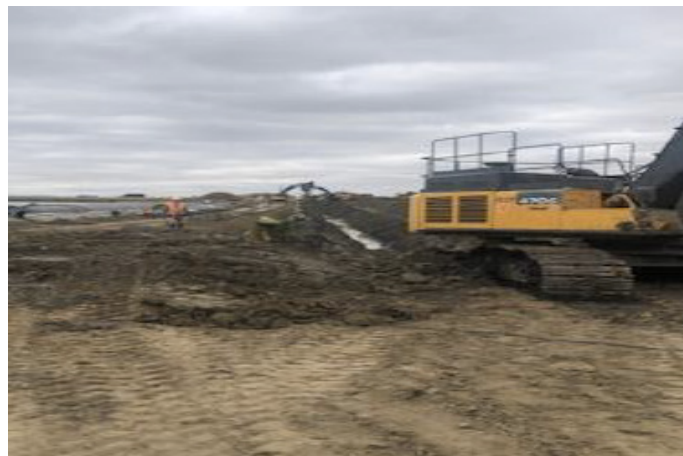
Digging ditch on east side of aqua dam – km 165+200 – Sept 14, 2018
