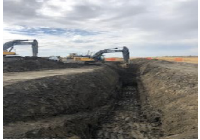
Digging bore bay – SF 124 –Sept 10, 2018
