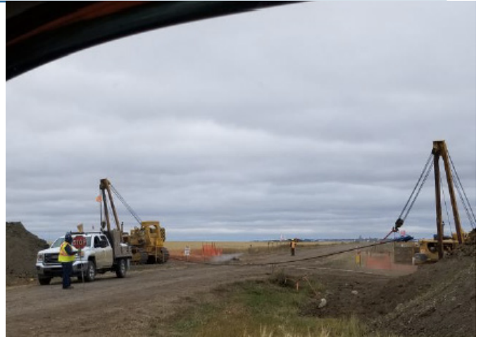
Equipment crossing with reach rod – km 149+936 – Sept 14, 2018
