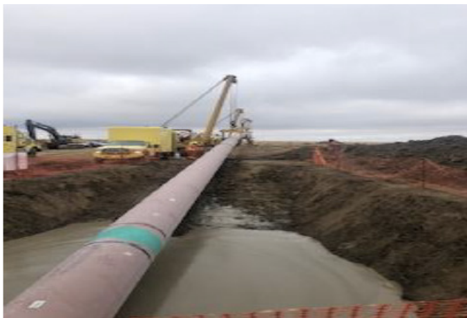
Bore section being pulled on west side of SF 107 – Sept 14, 2018
