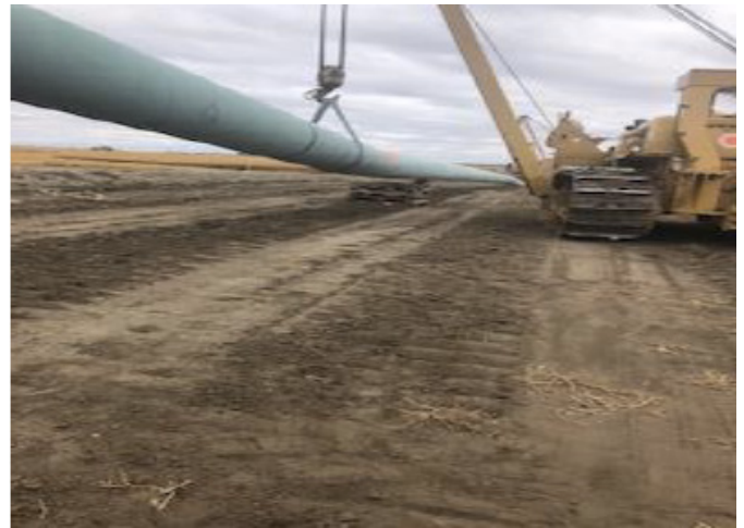
Aquadam about to be lifted and put into ditch – km 165+100 – Sept 14, 2018
