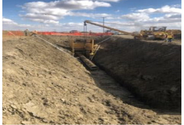
Trench box installed – SF 121 – Sept 11, 2018
