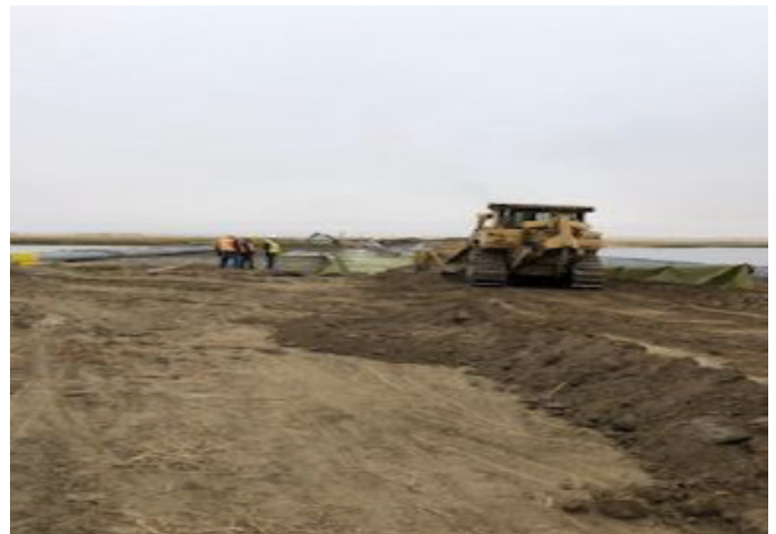
Crew building ramp across the wetland – km 165+200 – Sept 13, 2018
