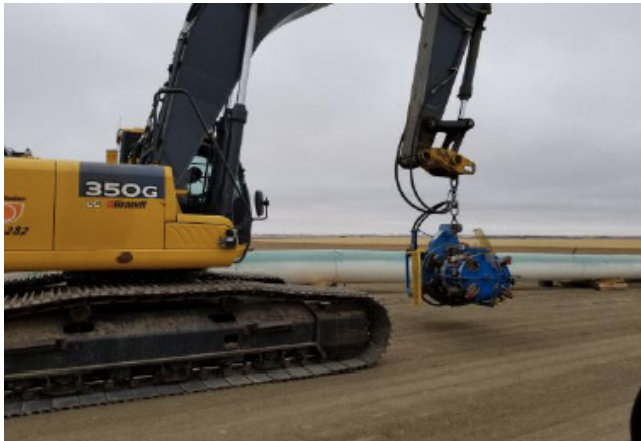
Prep crew - Km 148+ 700 – Sept 10, 2018
