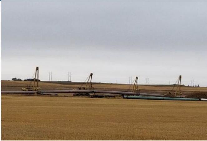
Booms prepping pipe – km 178+023 – Sept 13, 2018
