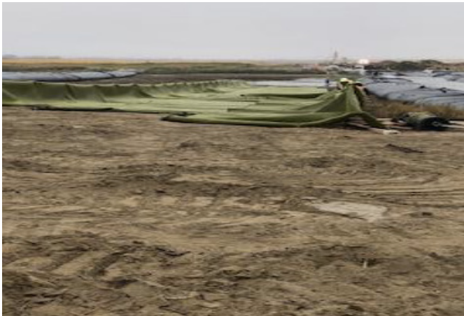
Geo tec for ramp access (aquadam) - km 165+100 – Sept 13, 2018
